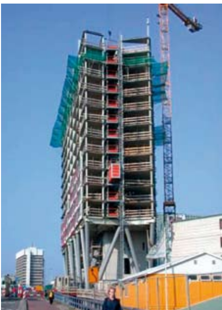
(Above) Building during construction
