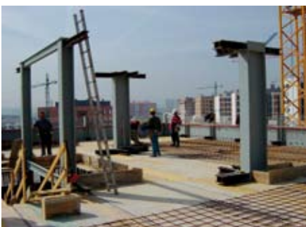
Floor with internal columns in the building works
