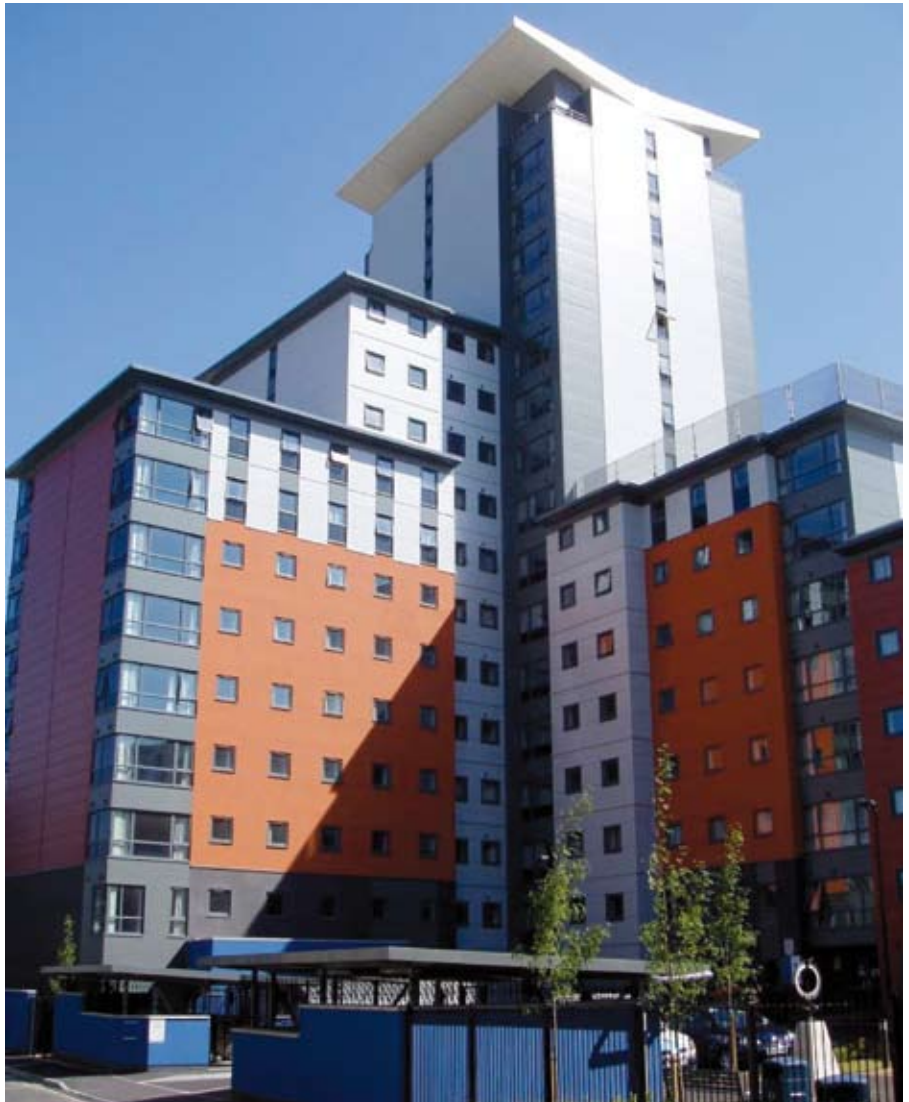
Figure 2.2 16-storey student residence constructed using a primary steel frame and light steel infill walls (Southampton, UK)
