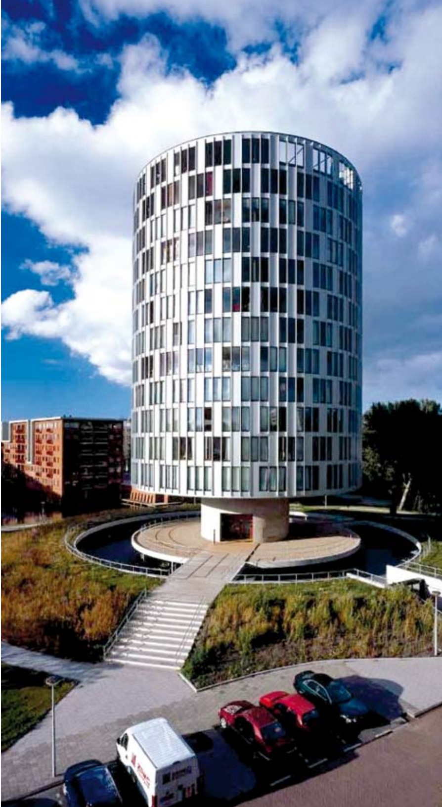
Figure 8.7 Multi-storey apartment building with a steel structure: Schutterstoren in Amsterdam.
