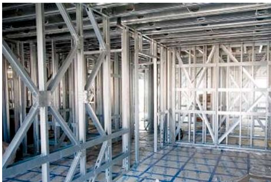
Figure 4.2 Platform construction of braced light steel wall in housing Fusion Building Systems
