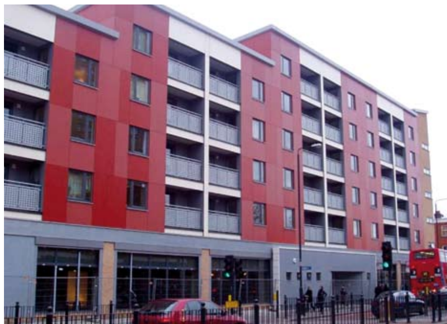
Figure 6.7 Completed modular building in Figure 6.6
