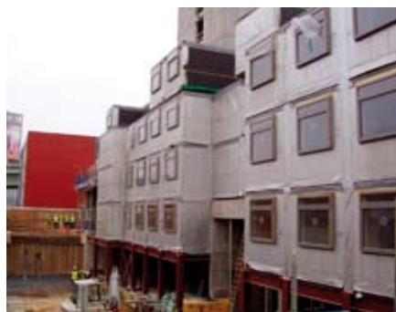
Installation of module on steel podium
