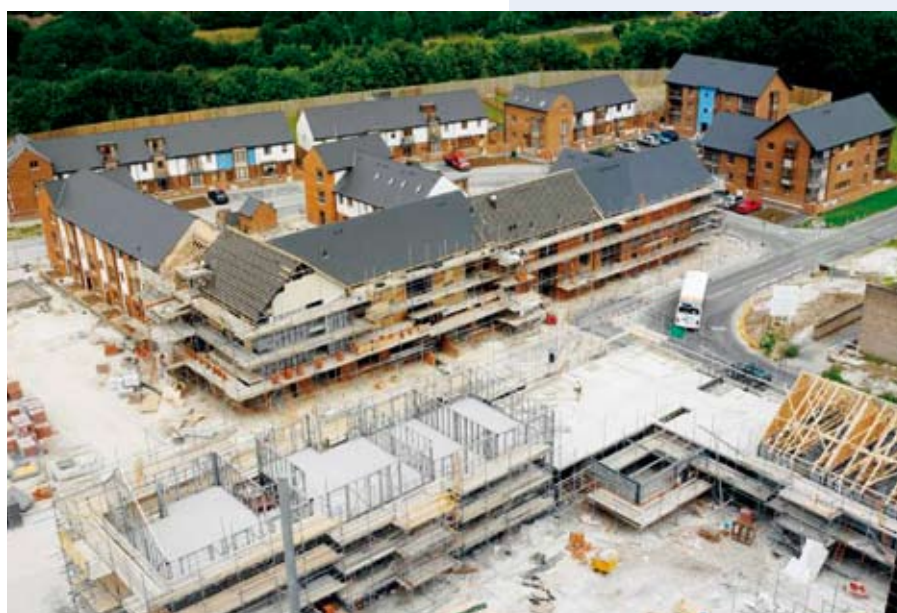
Figure 8.1 Housing project using light steel framing (Basingstoke) HTA Architects
