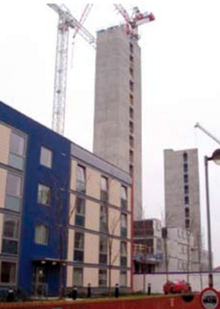
Modules attached to concrete core
