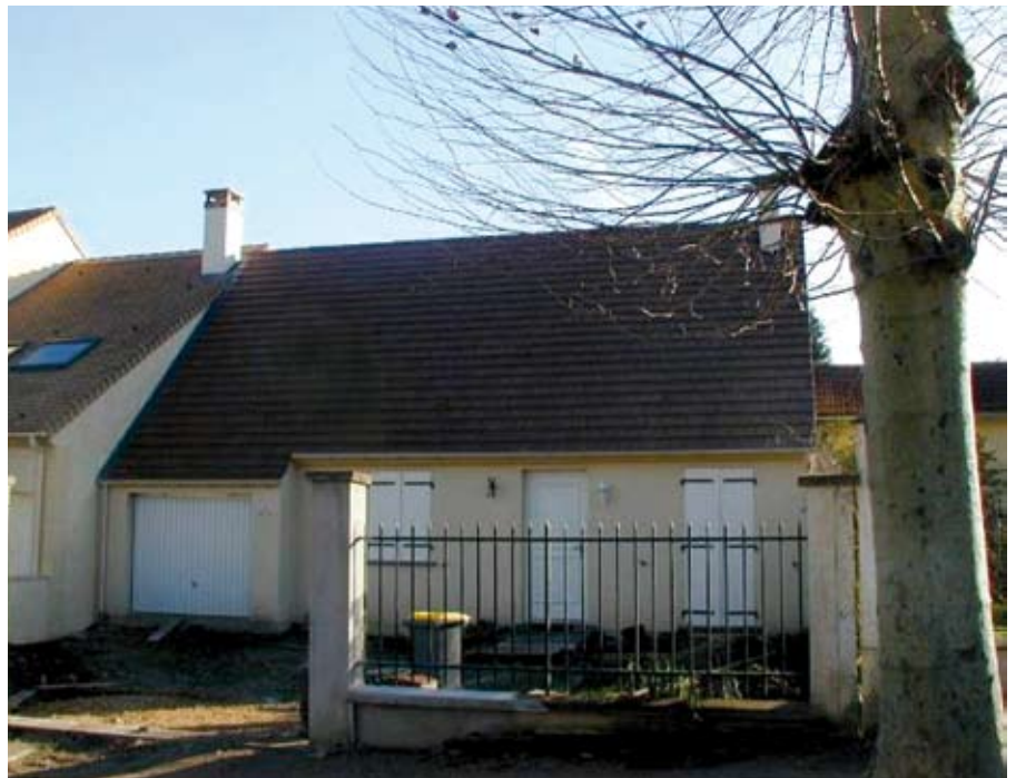
Figure 8.14 Maison Phénix during construction, showing the roof details for a single storey house
