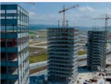
Bioclimatic Towers under construction
