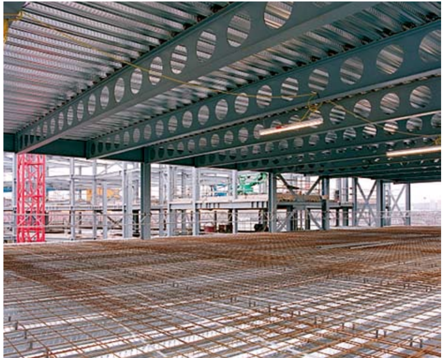
Figure 5.3 Composite steel decking and composite cellular beams
