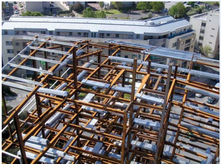
Figure 5.1 Steel frame using ASB sections and deep decking being installed
