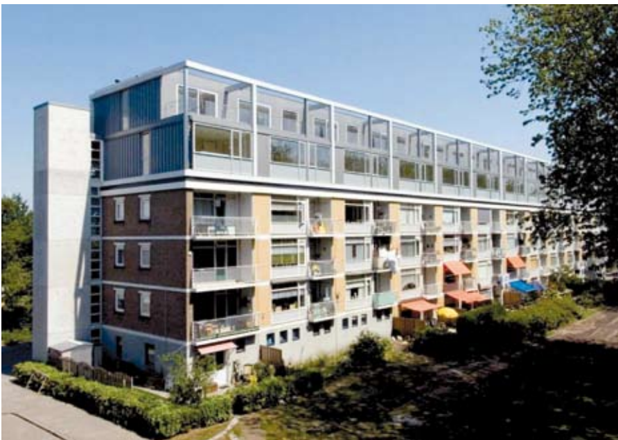
Figure 8.5 Roof-top extension with maisonettes: Het Lage Land in Rotterdam
