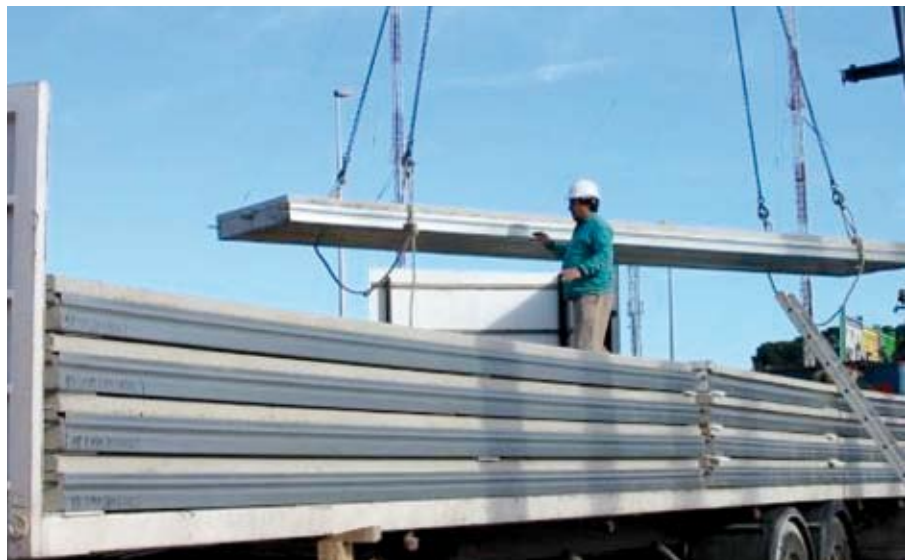
Figure 8.13 Cofradal lightweight slab units – typical cross section and panels during installation
