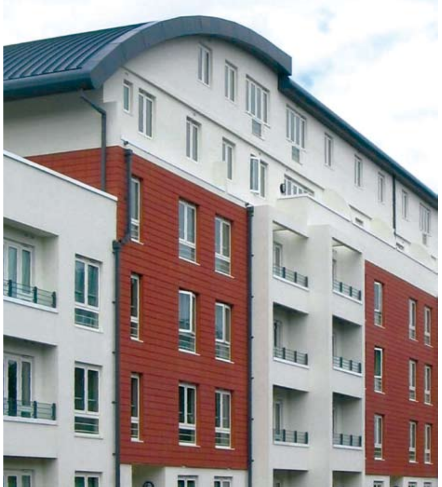
Figure 7.2 Insulated render combined with clay tiles attached to light steel infill walls
