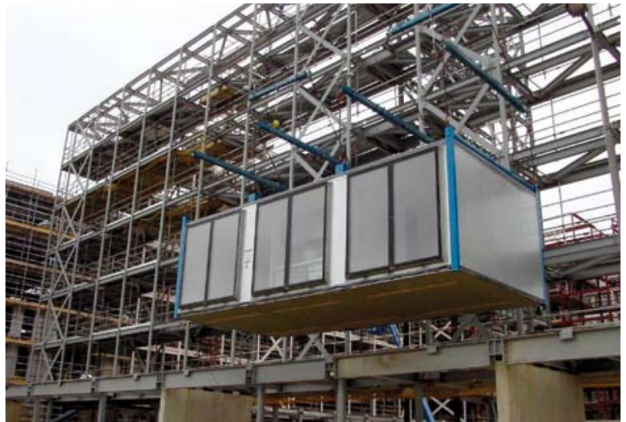
Figure 8.3 Steel external framework combined with highly glazed modules, MOHO, Manchester Yorkon and Shed KM Architects
