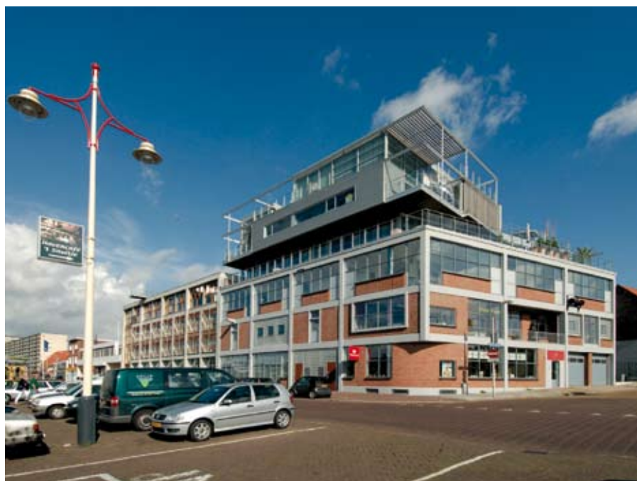
Figure 8.6 Transformation of an old warehouse with a spectacular view: Nautilus & IJsviss in The Hague (Winner National Steel Prize 2006, category Residential buildings).
