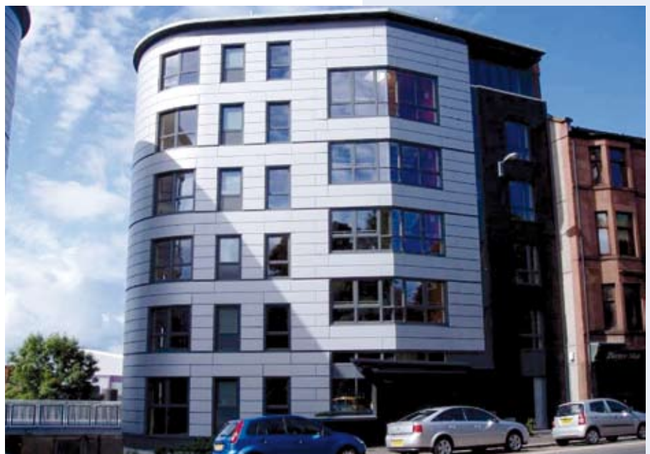
Figure 7.1 Residential building in light steel framing and with metallic cladding in Glasgow Peck and Reid Architects & Metsec
