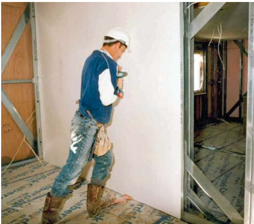
Figure 4.6 Plasterboard being attached to separating wall at X bracing
