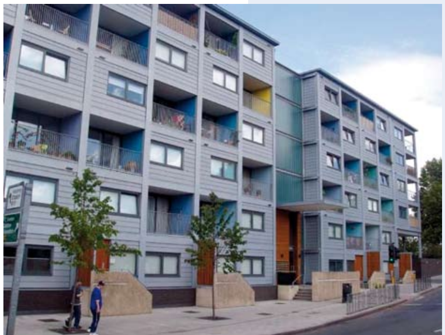
Figure 6.1 Modular residential building with integral balconies, London AHMA Architects & Yorkon
