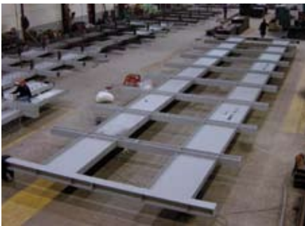
Off-site fabrication of the façade structural panels
