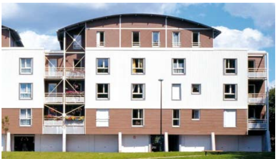
Figure 2.3 Steel-framed apartment building in Evreux, France with light steel walls and floor decking and lightweight cladding Architects: Dubosc & Landowski
